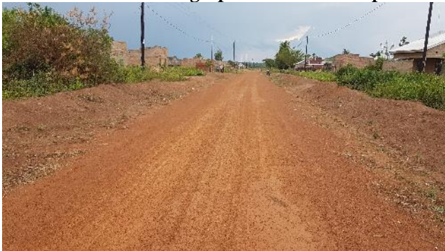
Ch. 0+000: Gravelled road surface
