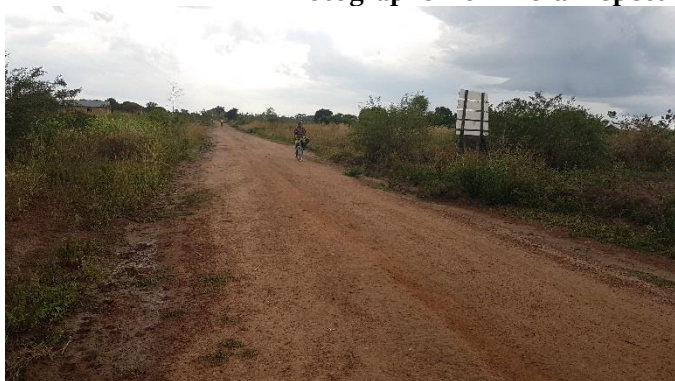
Shaped sections of the road
