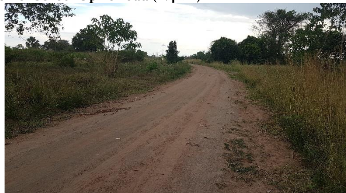
Shaped sections of the road
