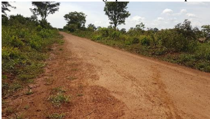
0+000: Shaped section of the road
