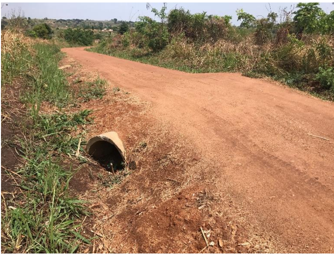
Ch. 2+200: Culvert installation without end structures
