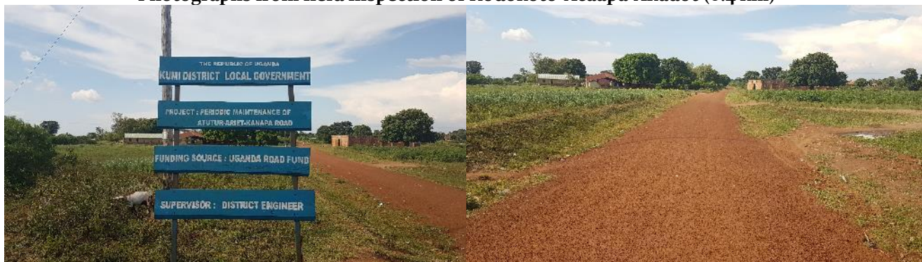
Ch. 0+000: Project profile board lacking the financial year Ch. 0+200: Gravelled sections
