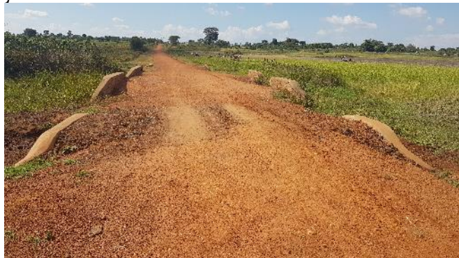
Ch. 6+200: Inferior backfill material for culverts
