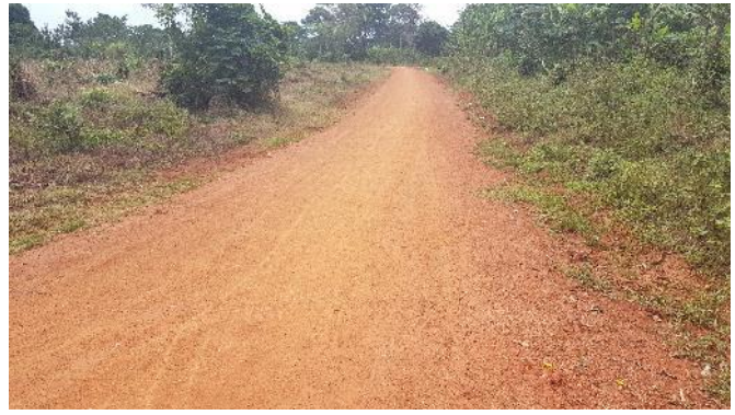
Ch. 0+850: Gravelled sections
