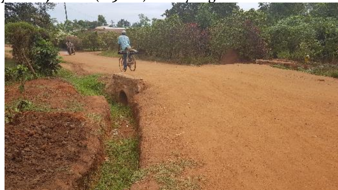
Ch. 0+000: Drainage improvements
