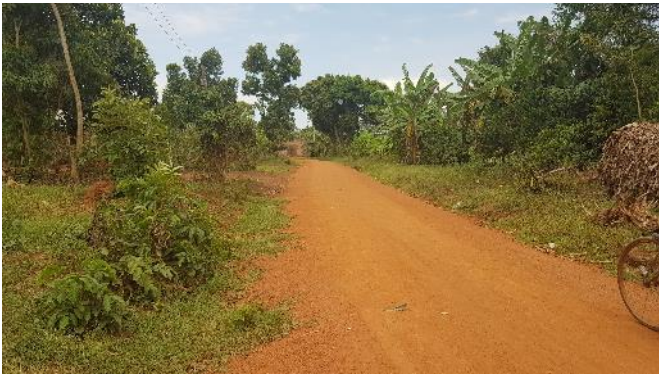
Ch. 0+380: Gravelled sections
