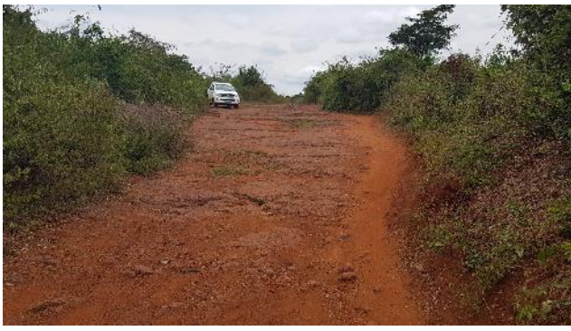
Ch. 31+900: Rock outcrop requiring gravel filling
