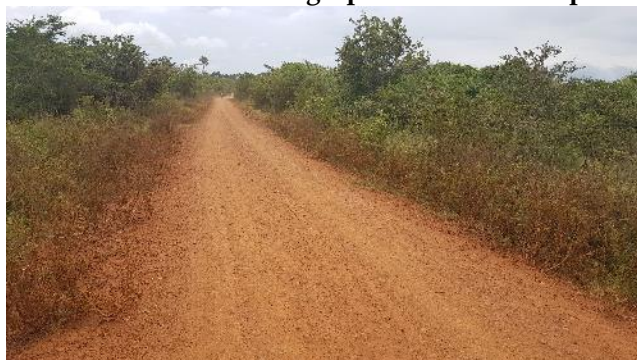
Ch. 4+100: Gravelled section with inadequate RMM
