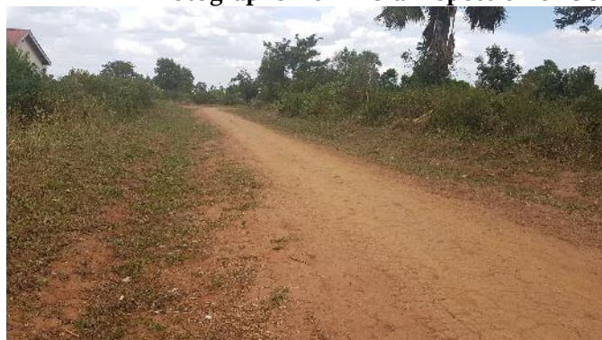
Opened section of the road
