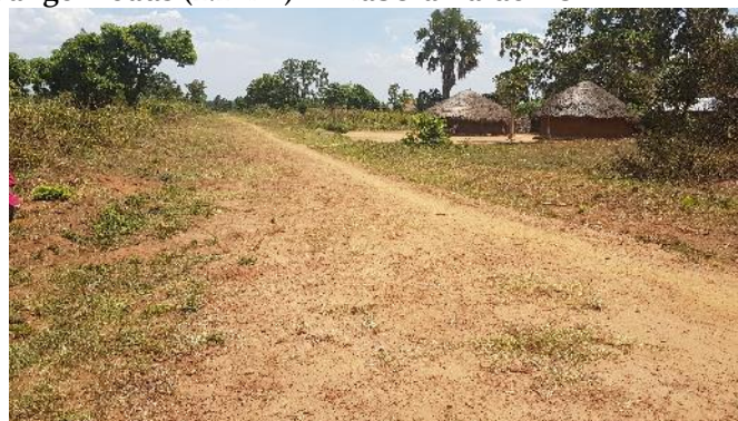
Narrow carriageway due to lack of vehicular traffic and RMM
